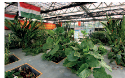
The Chinese City of Shenzen uses Hungarian technology to perform biological sewer treatment.
